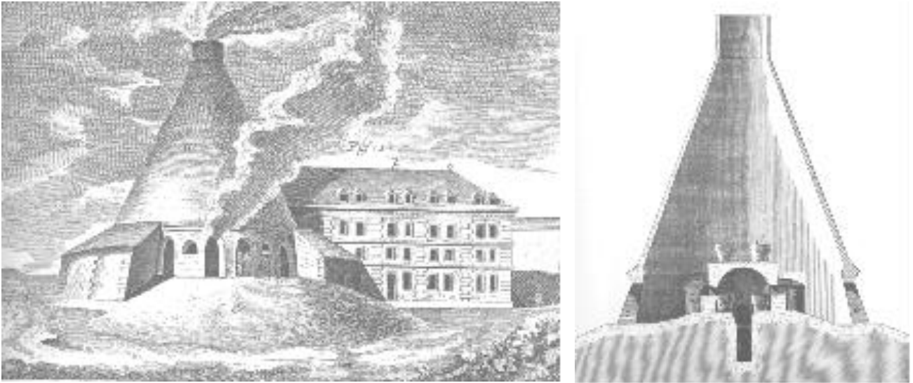
Fig. 3. Mid-18 th century English glass house with external furnace. (10)
